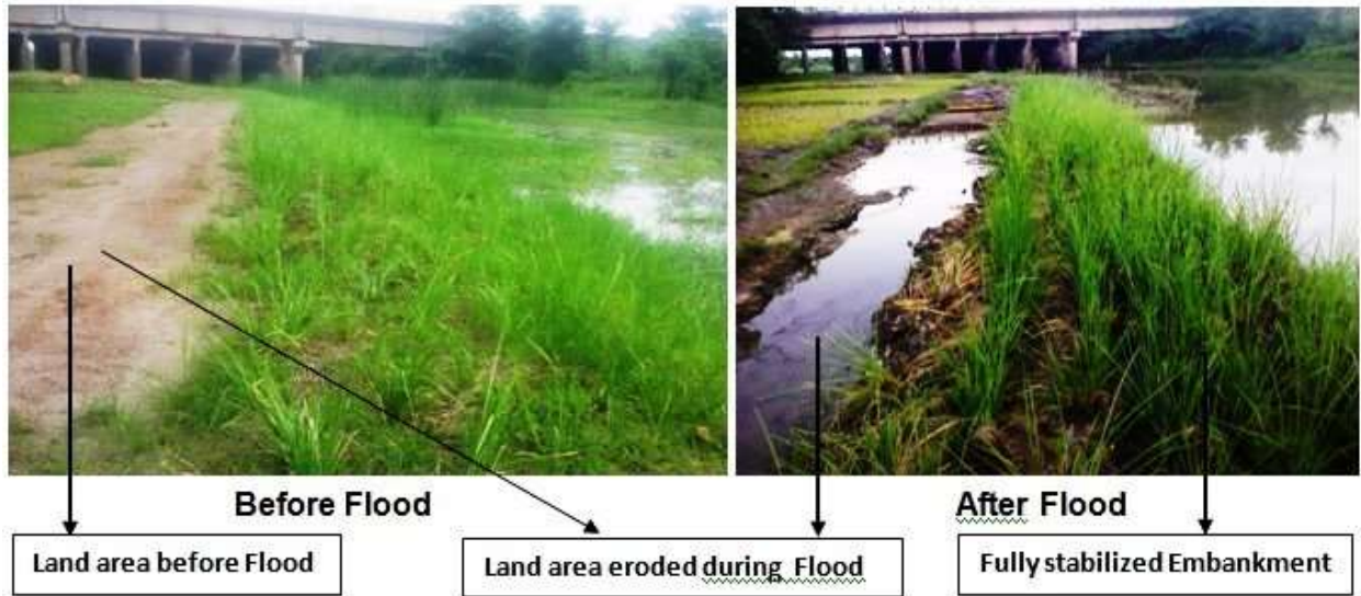
Stabilized River Embankment
